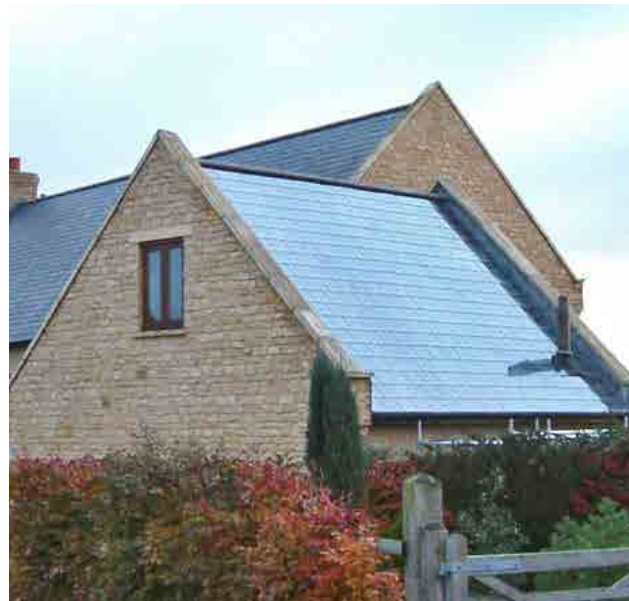
Figure 80: Example of solar tiles integrated into the roof from the outset.
