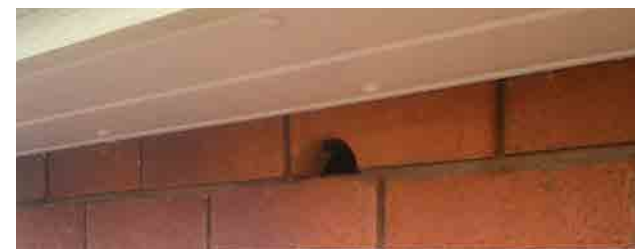
Figure 76: Example of a swift brick under an eave.
