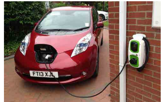
Figure 51: Example of off-road mounted car charging points.
